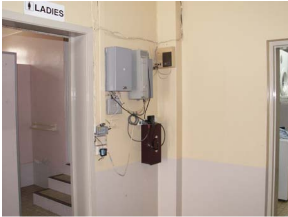
Figure 2. South-east corner main appliance bay.
