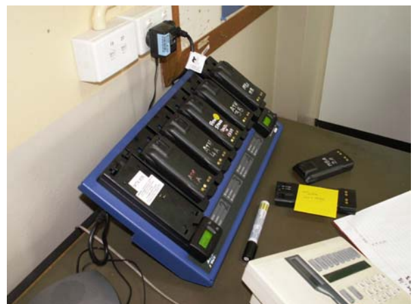
Figure 6. Main office, radio battery charger on desk.
